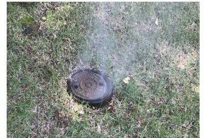
The smoke should not enter your home or business if it is properly plumbed, vented, and the water traps contain water. If smoke does enter a home or building, it will clear within 30 minutes with proper ventilation.
